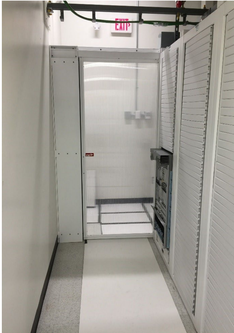
Figure 3 - Blanking Panels And Sliding Containment Door
