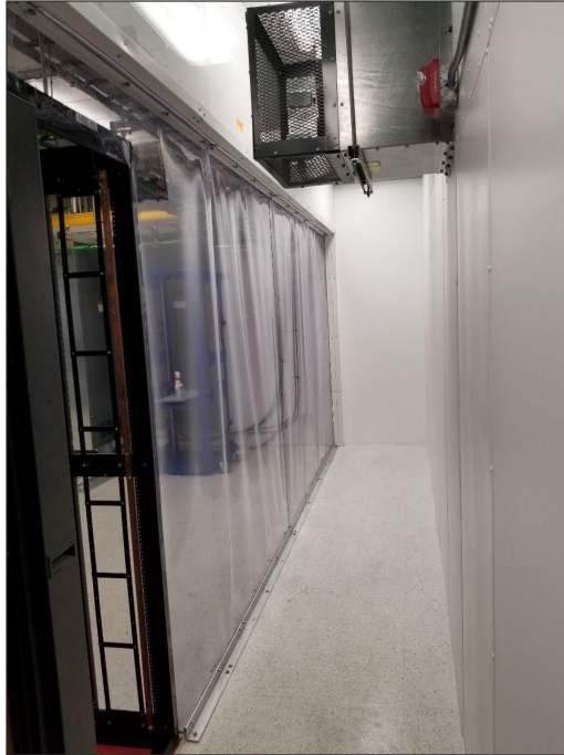
Figure 4 - Airflow Containment With Curtains
