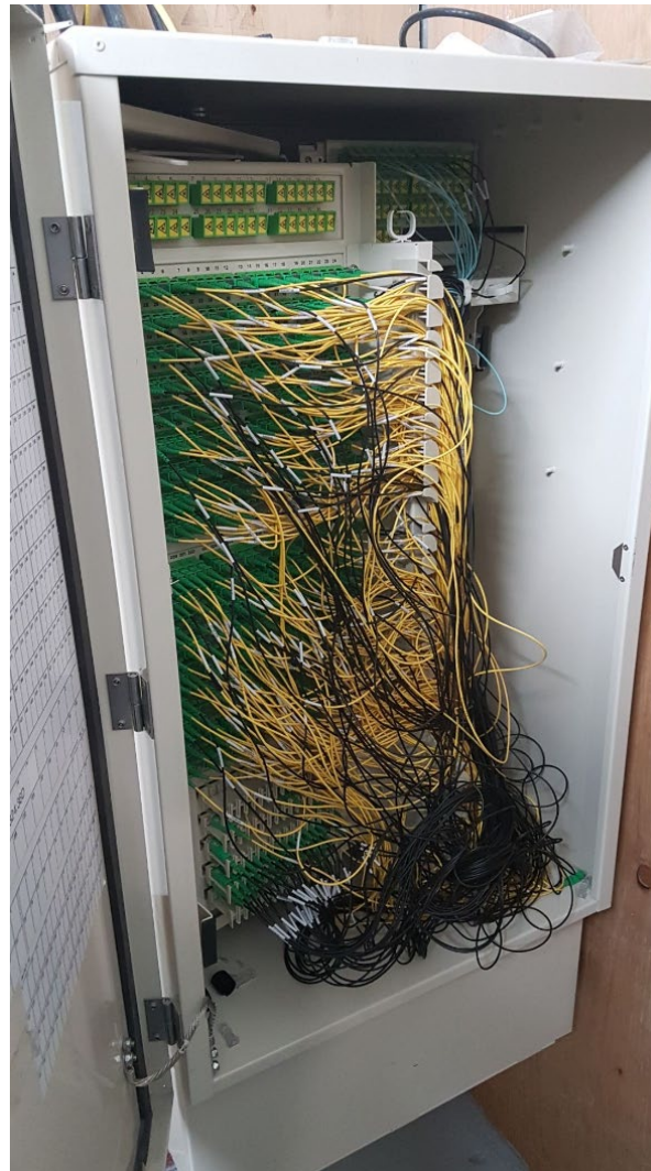
Figure 4 - FTC with Active Drop Configuration
