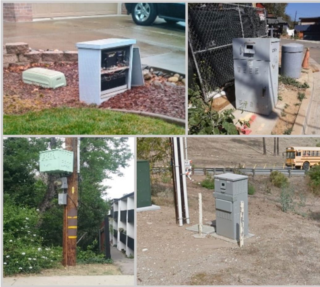
Figure 2 - Example cable broadband powering sites. The variability in available space, loading, and local regulations makes a one-size-fits-all solution for ESS solutions nearly impossible.
