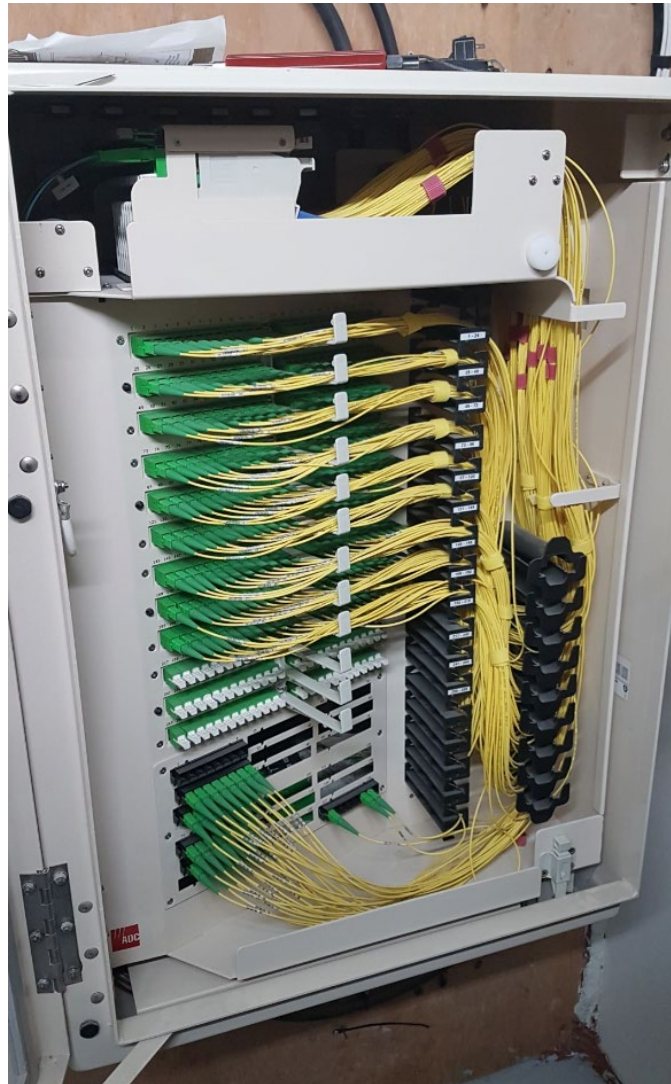
Figure 16 - FTC with Hot Drop Configuration
