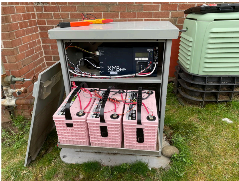
Figure 3 – Pad mounted Outside Plant with Batteries Shown
