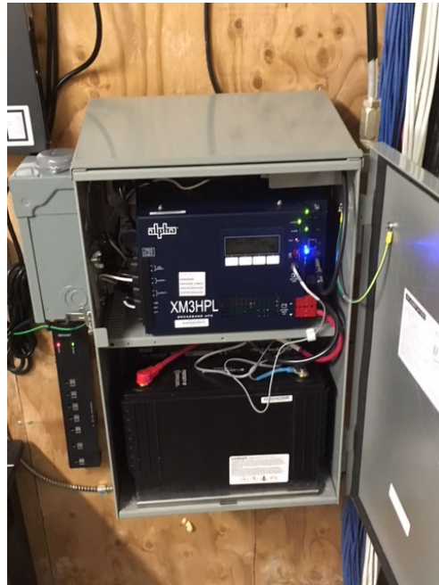
Figure 10 – Small Broadband UPS for Dedicated R-OLT Powering
