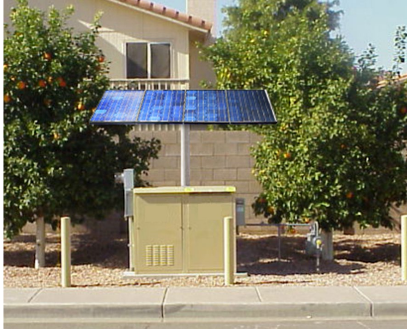
Figure 11 - Example of a solar augmented cable power supply
