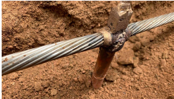
Figure 1 – Exterior Ground Ring Conductor Exothermically Welded To A Ground Rod
