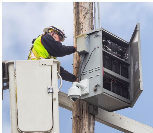
Figure 8 – Typical Broadband UPS
