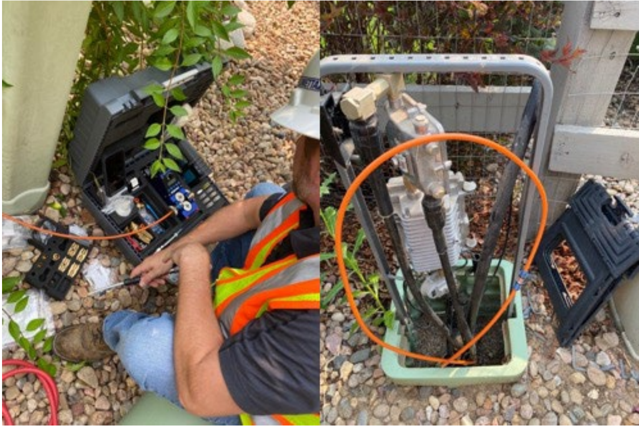
Figure 11 – Location # 2 Left: Blowing of fiber, Right: Conduit spliced in ped for blowing continuity
