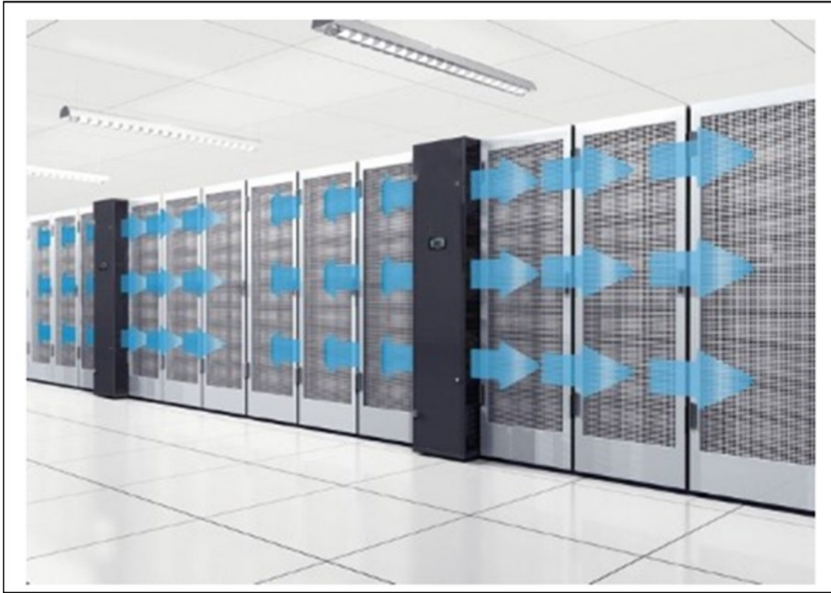
Figure 4 - Example of in-row cooling where air conditioning units fit inside rack rows. Courtesy: PRWeb
