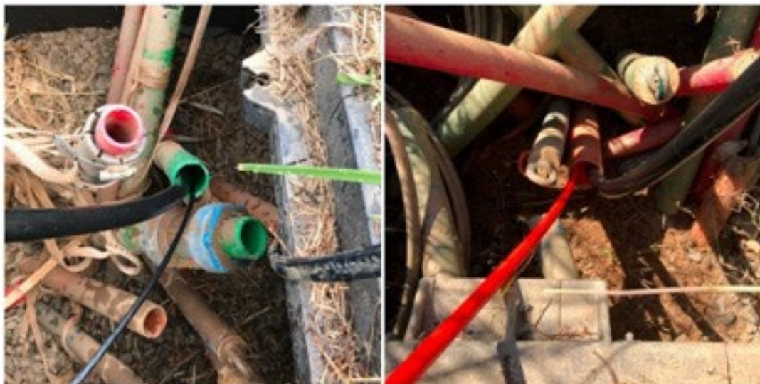
Figure 8 – Finished micro-fiber and micro-duct installed
