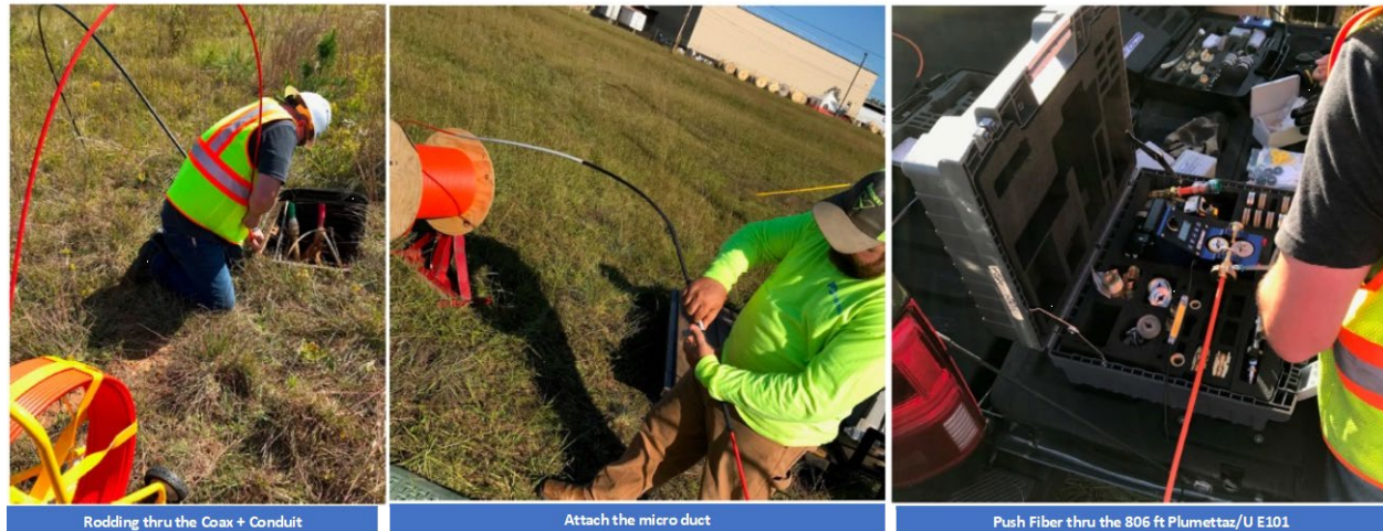
Figure 7 – Illustrating the Rod-and-Rope process and blowing fiber into the installed micro-duct
