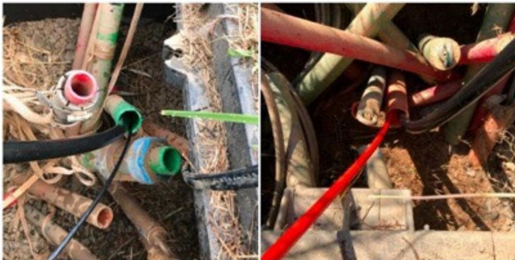
**Figure 8 – Finished micro-fiber and micro-duct installed**
