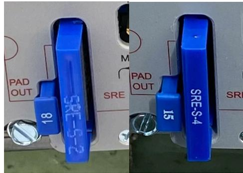
**Figure 12 – Sub-split return equalizers installed in mid-split amplifiers**
