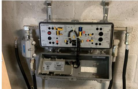
**Figure 11 – Sub-split amplifier installed in a mid-split system**
