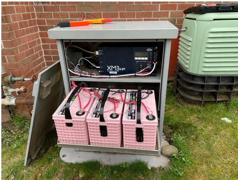
**Figure 3 – Pad mounted Outside Plant with Batteries Shown**
