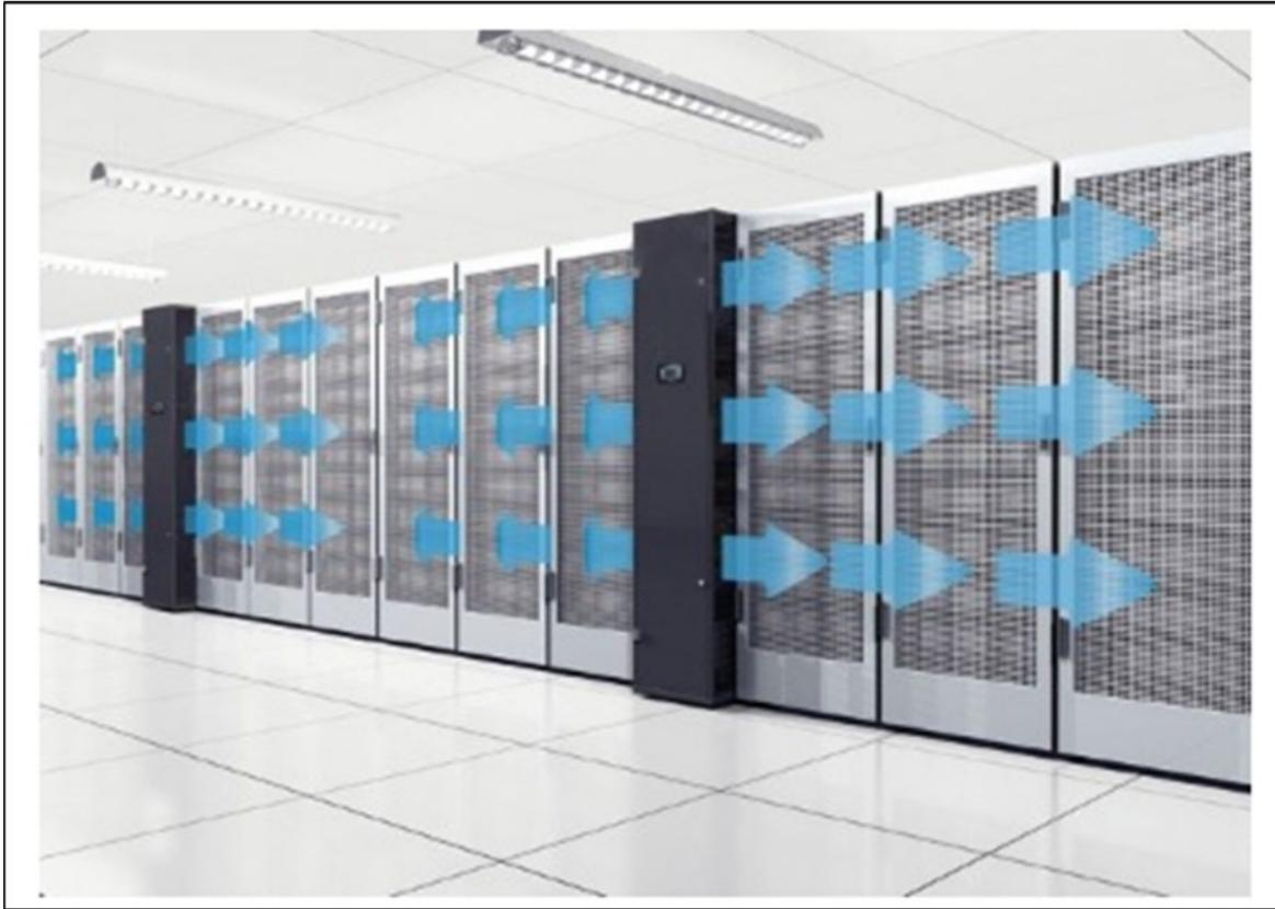
**Figure 4 - Example of in-row cooling where air conditioning units fit inside rack rows.
