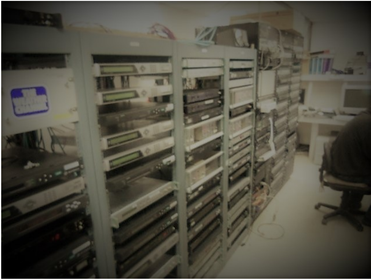
Figure 2: An analog-only two-way Headend. Image by Author. Circa 12/2018
