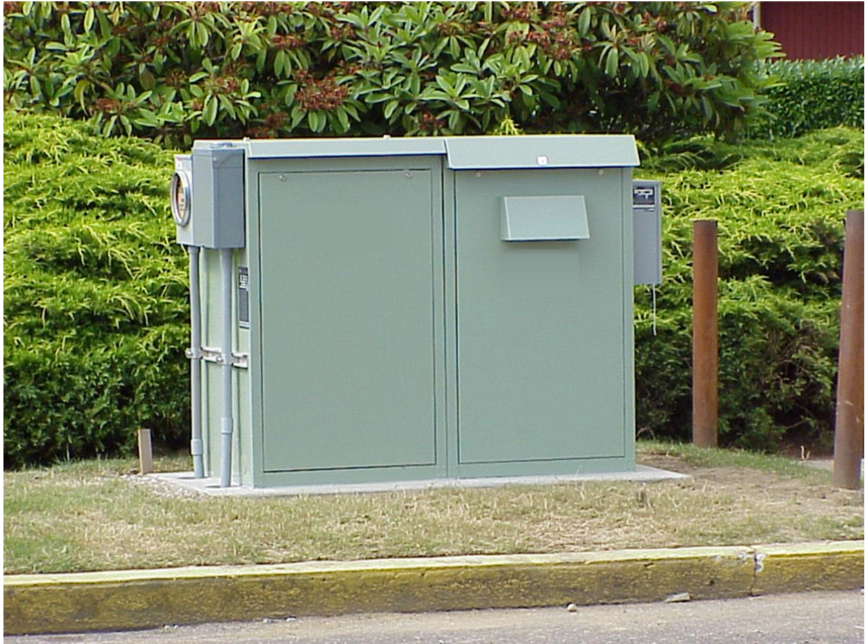
Figure 3 - Typical Curbside Generator Installation Using Natural Gas
