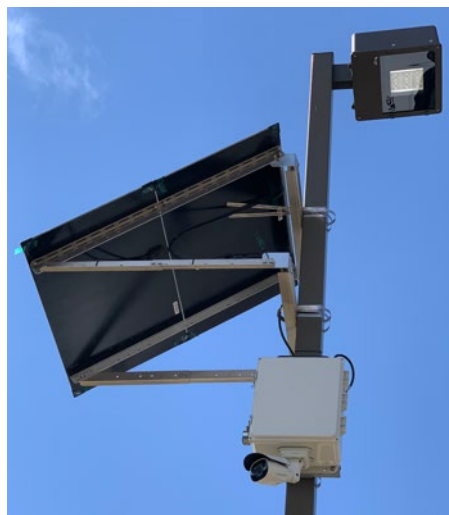
Figure 9 - Example of outdoor LPR install
