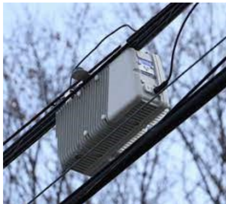
Figure 5 - Small Cell Radio within Communications Space 20
