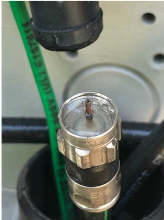
Figure 20 - Water coming out of the end of the connector at the ground block
