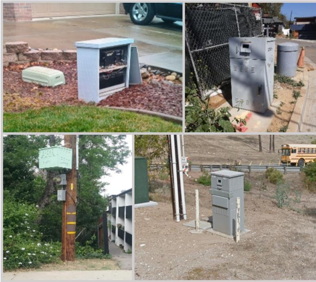
Figure 1 - Example cable broadband powering sites. The variability in available space, loading, and local regulations makes a one-size-fits-all solution for extended run time nearly impossible.
