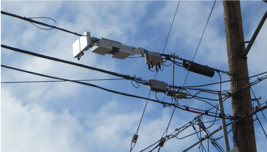
Figure 14 - Remote Line-Powered Small Cell
