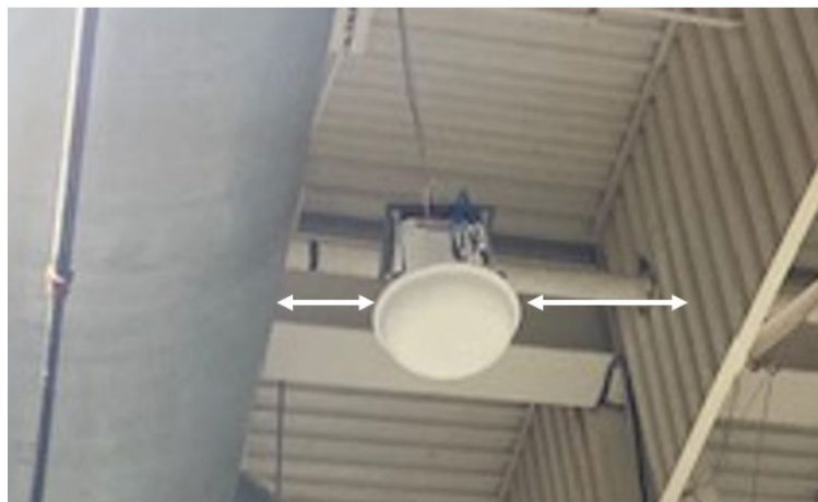
Figure 10 - Antenna blocked by metal duct and rail
