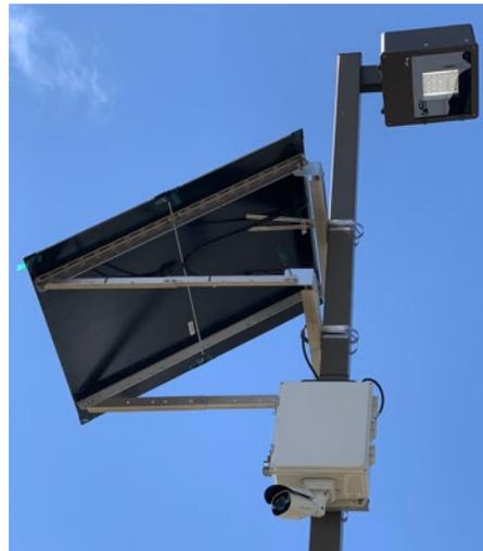
Figure 9 - Example of outdoor LPR install
