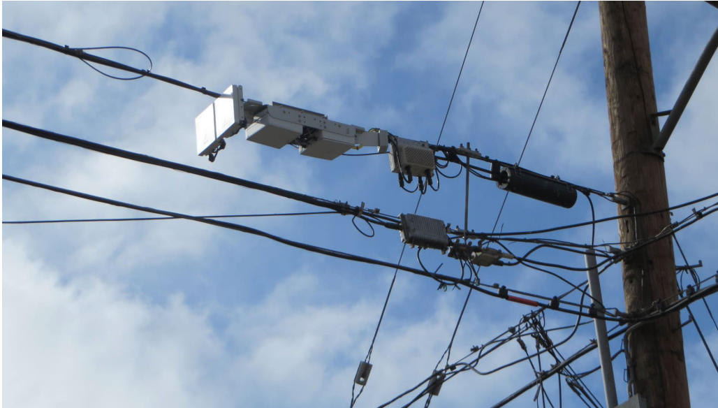
Figure 14 - Remote Line-Powered Small Cell
