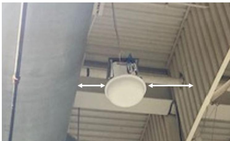
**Figure 10 - Antenna blocked by metal duct and rail**
