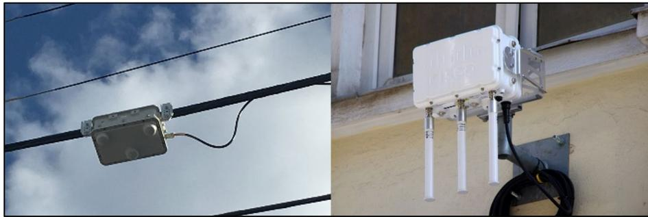
**Figure 2 – Service Provider Wi-Fi Access Points**
