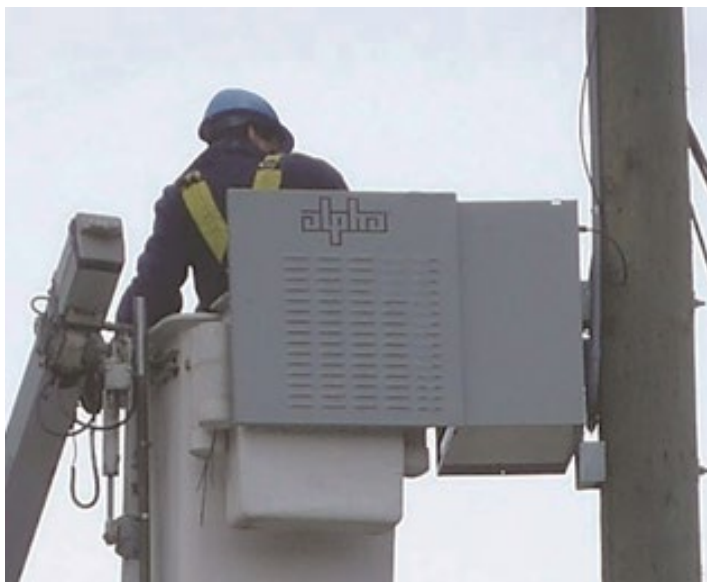
Figure 6 – Typical Pole Mounted Broadband UPS
