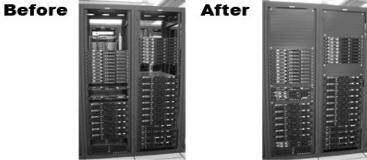
Figure 9 - Open RUs On Left, PlenaForm Systems Blanking Panels Installed On Right
