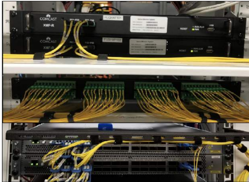
Figure 8 – Actual Comcast Installation of the Continuous Pervasive Monitor
