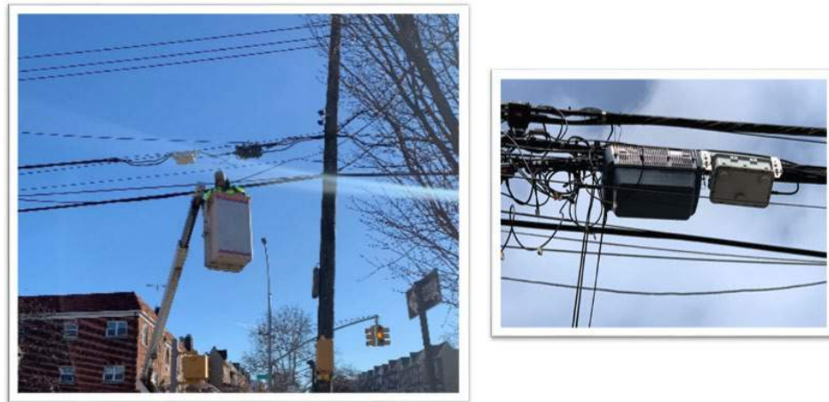
Figure 5 Strand Mount Outdoor Deployment
