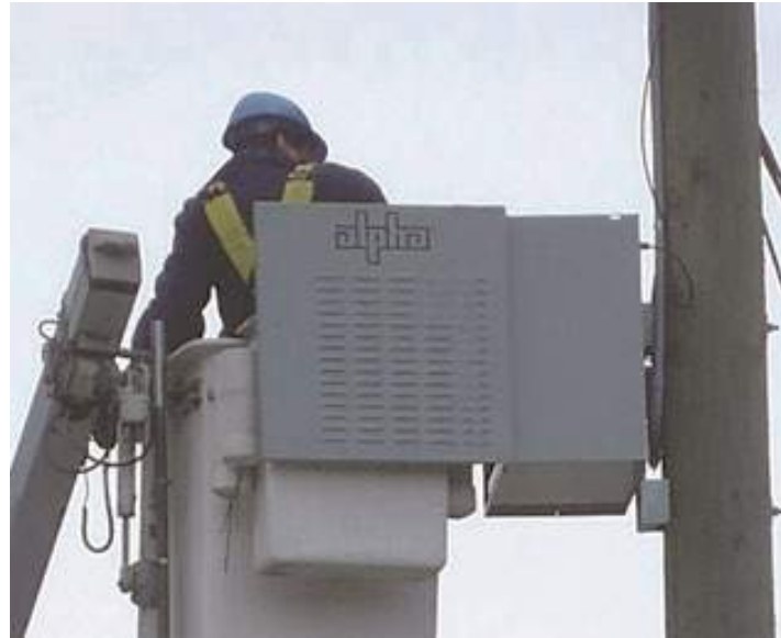
Figure 6 – Typical Pole Mounted Broadband UPS
