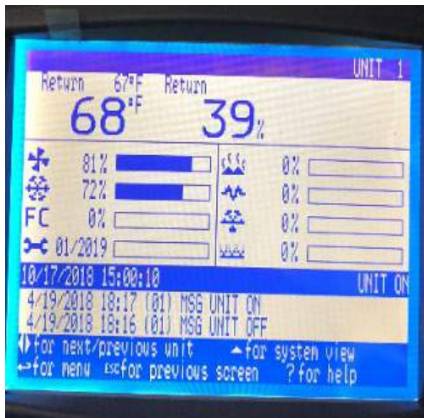
Figure 8 - Vertiv Performance And Set Point Display With Function Key
