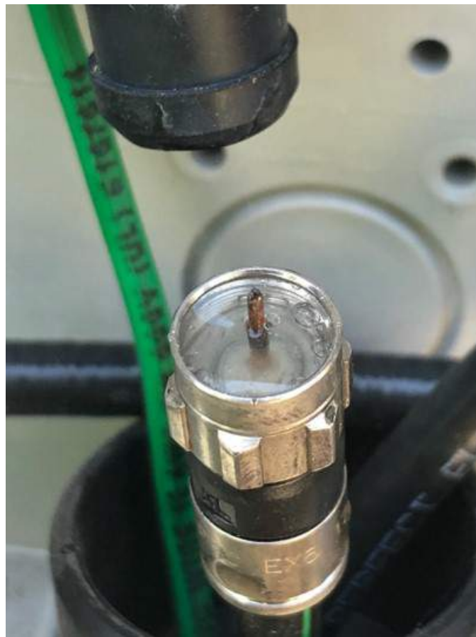
Figure 23. Water coming out of the end of the connector at the ground block.
