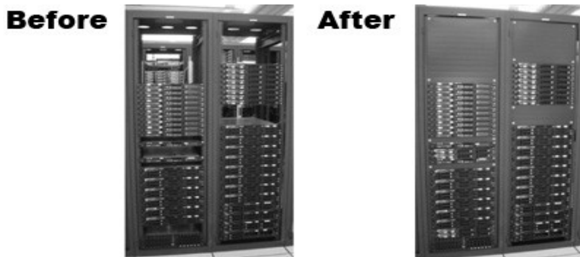
Figure 9 - Open RUs On Left, PlenaForm Systems Blanking Panels Installed On Right
