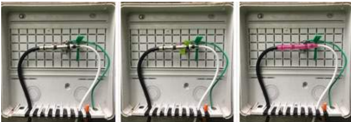
Figure 2 - Image example of House Box category; panels 2 and 3 highlight the bond block and filter, respectively
