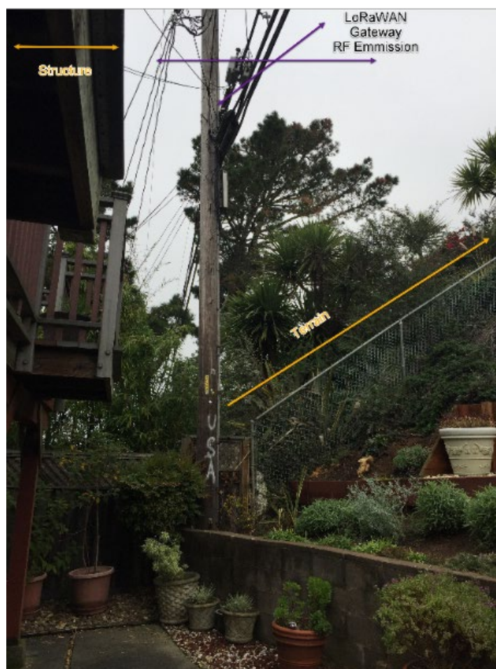
Figure 25 HFC Based questionable deployment RF blocked by terrain and structure.
