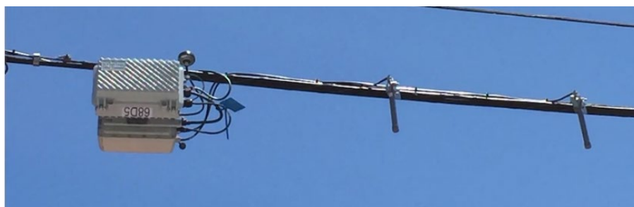
Figure 21 HFC deployed LoRaWAN Gateway and Antennas
