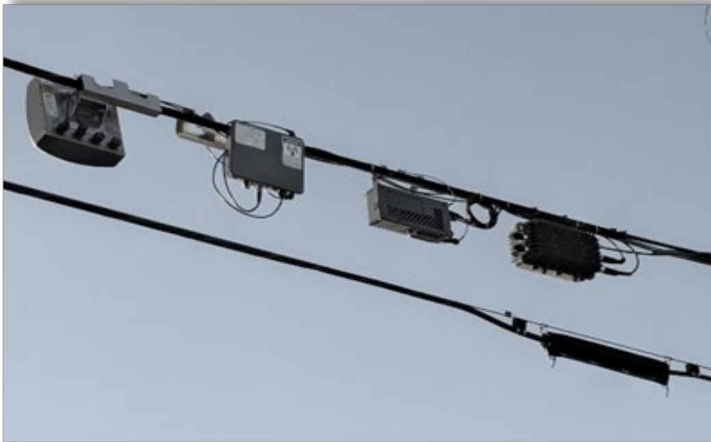
Figure 6 - An example of current strand-mount DAA applications housings
