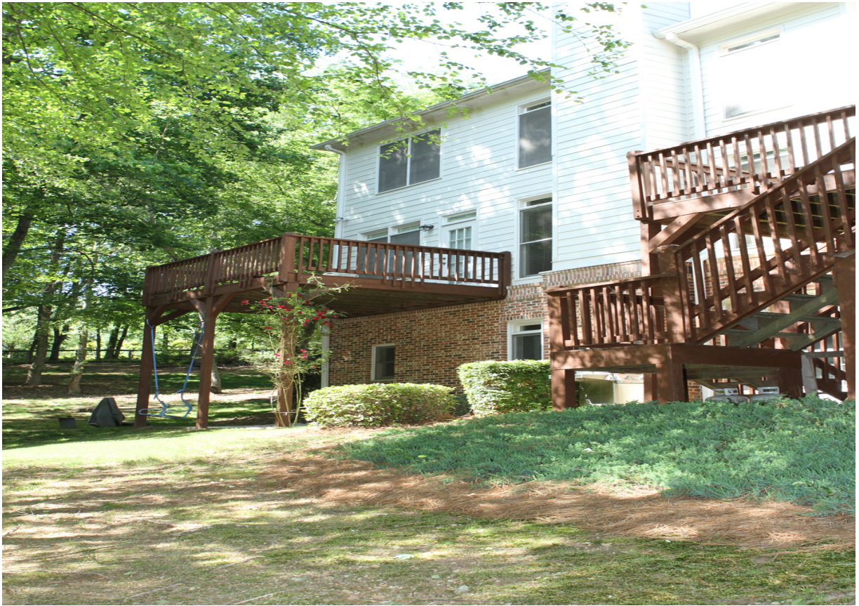
Figure 5 – WiFi test house, rear view
