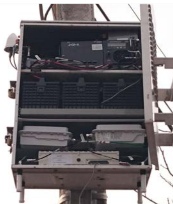
Figure 7 - Enclosure with Wireless Equipment
