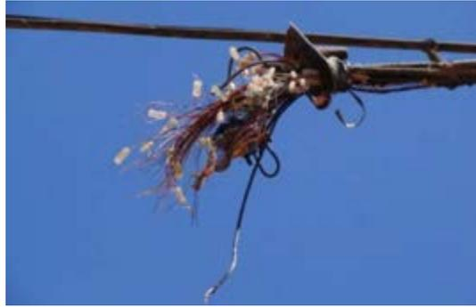
**Figure 2 – Photo of a Stolen Optical Unit, Optical and Copper Cables in a Yarn String**
