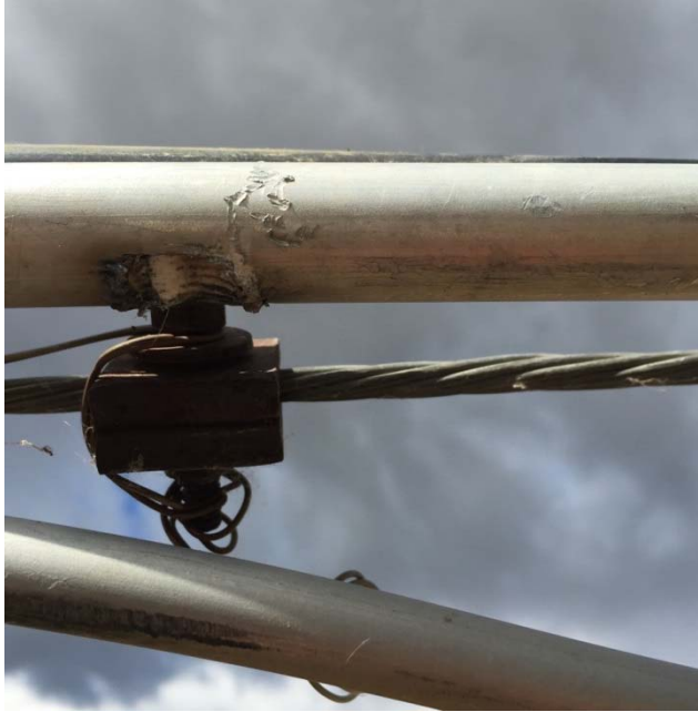
Figure 9. A hole was rubbed through a hardline coax shield causing UHF leakage.
