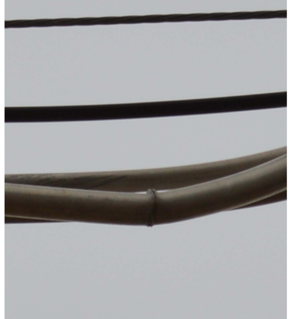
Figure 11. This is a radial crack that was not producing a VHF leakage alarm. After repair, signal quality improved for homes fed by this cable.
