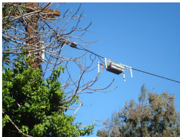
Figure 5: Strand Pico Cell in service
