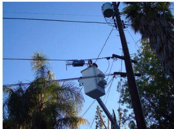
Figure 4: Installing a Pico Cell
