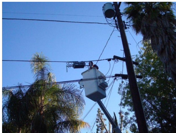
Figure 4: Installing a Pico Cell
