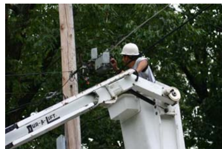
Figure 1 Wi-Fi Microcell being installed on HFC
