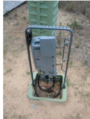
Figure 16 Pedestal mounted BTS
