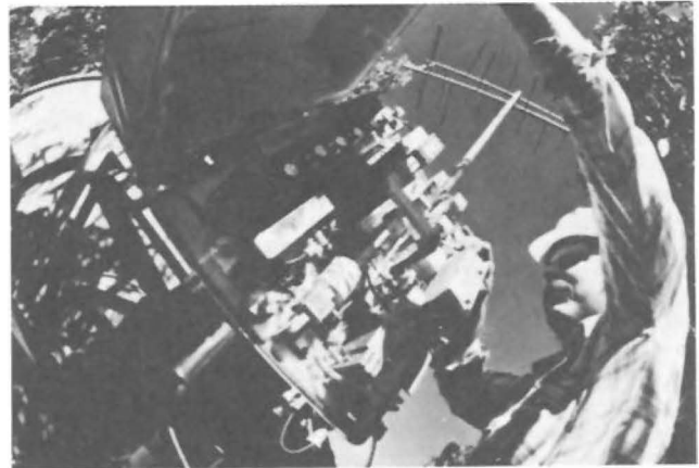
Figure 1 Typical CATV system AML hub.
