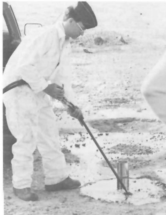
Fig. 2 - Air Force technician floods a debris-filled bomb crater with reactive PERCOL mixture, which gels in two minutes and cures in 30 minutes.
