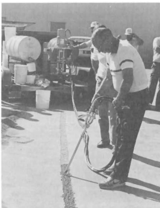
Fig. 18 - Reactive PERCOL mixture flows out of nozzle into trench, percolating through the aggregate and encapsulating the cable.
