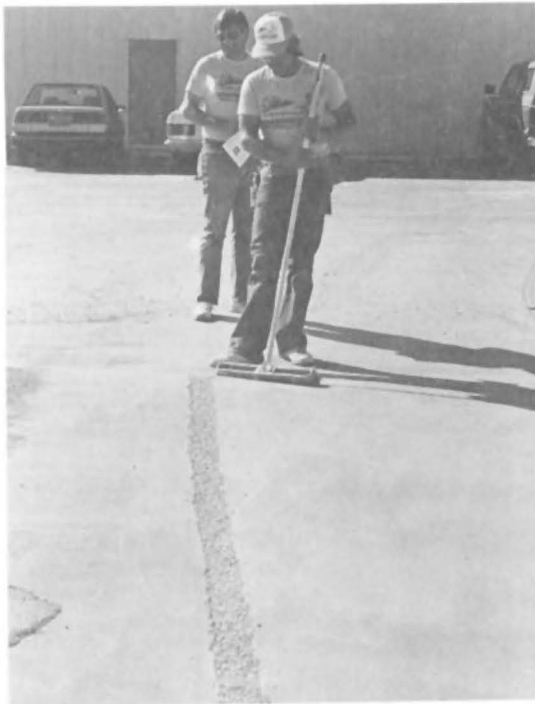
Fig. 16 - Asphalt pavement debris from saw cut is swept back into trench, supplemented by washed, dry pea gravel, cold mix, or recycled asphalt.
