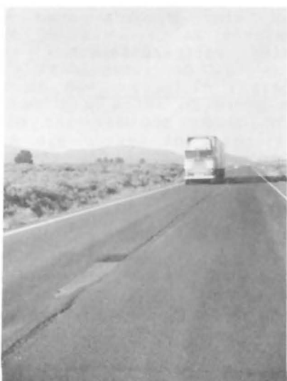
Fig. 3 - Crater (near center line) on U.S. 97 repaired with PERCOL and rock aggregate by California Department of Transportation.
