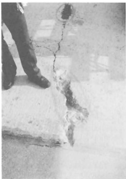
Fig. 6 - Fractured concrete pot-hole on aircraft runway which has been jack-hammered back to solid concrete.
