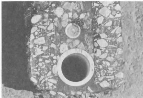
Fig. 21 - Showing how cables can be double-decked by repeating the PERCOL process in two stages.
