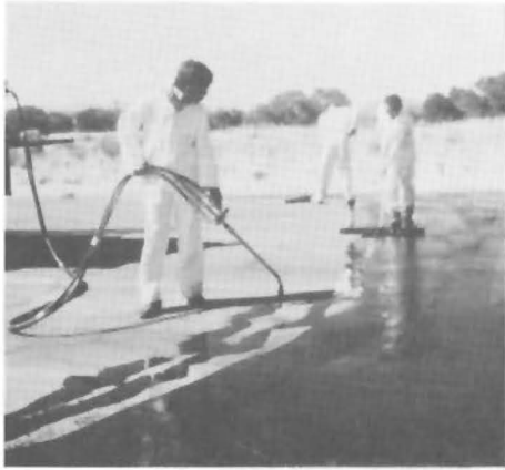
Fig. 10 - PERCOL reactive liquid is squeegeed over the surface of a deteriorated model airplane runway.
