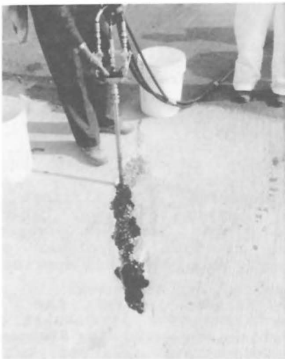
Fig. 8 - Aggregate filled cavity is flooded with reactive PERCOL polymer.
