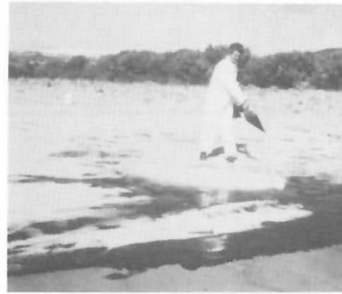
Fig. 11 - Broadcasting sand over the reactive PERCOL mixture before gelation.
