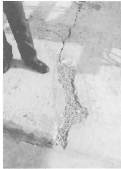
Fig. 7 - The cavity is filled with coarse, dry aggregate.
