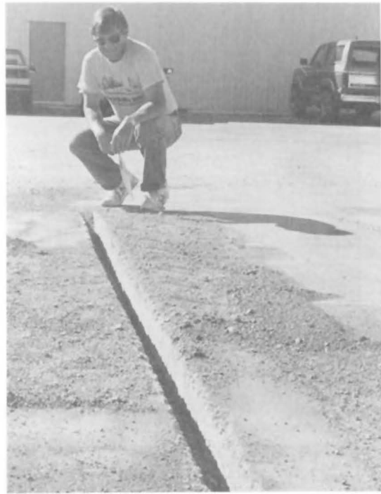
Fig. 15 - Trench sawed in asphalt pavement in which cable will be laid.
