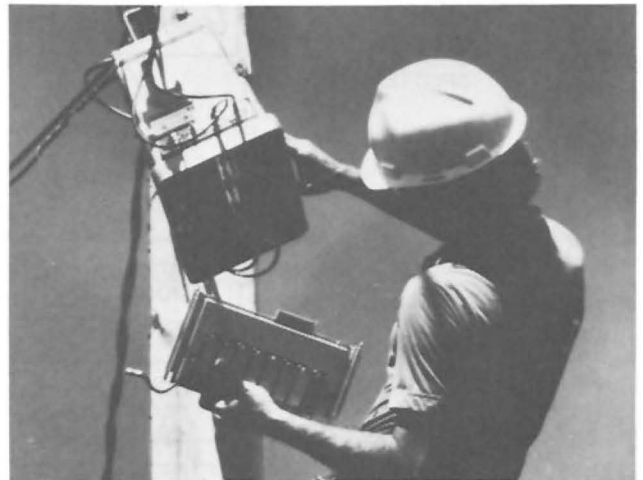
Fig. 1 OTAS Subscriber Terminal Each terminal has the ability to control seven (7) premium tiers plus basic on/off service per subscriber.
