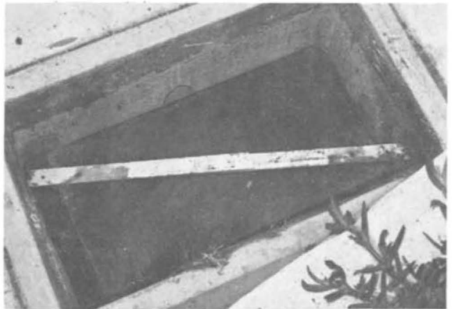
Figure 16. Use of liner in underground vault to provide air trap to protect distribution equipment from water.
