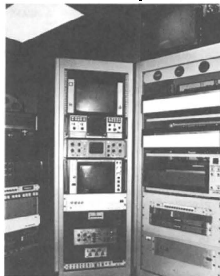
Fig. 7. Recording control and monitoring in center, camera control at left. At right, two of twelve recorders and quality-control player.
