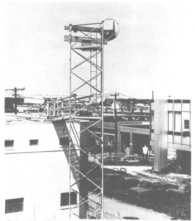
The Laser Link cableless CATV transmitting-receiving terminal in Garden City, NY incorporates quasi laser link concept of antenna and parabollic reflector equipment at top. Back view shows transmitter housing containing modulation and amplification components.
