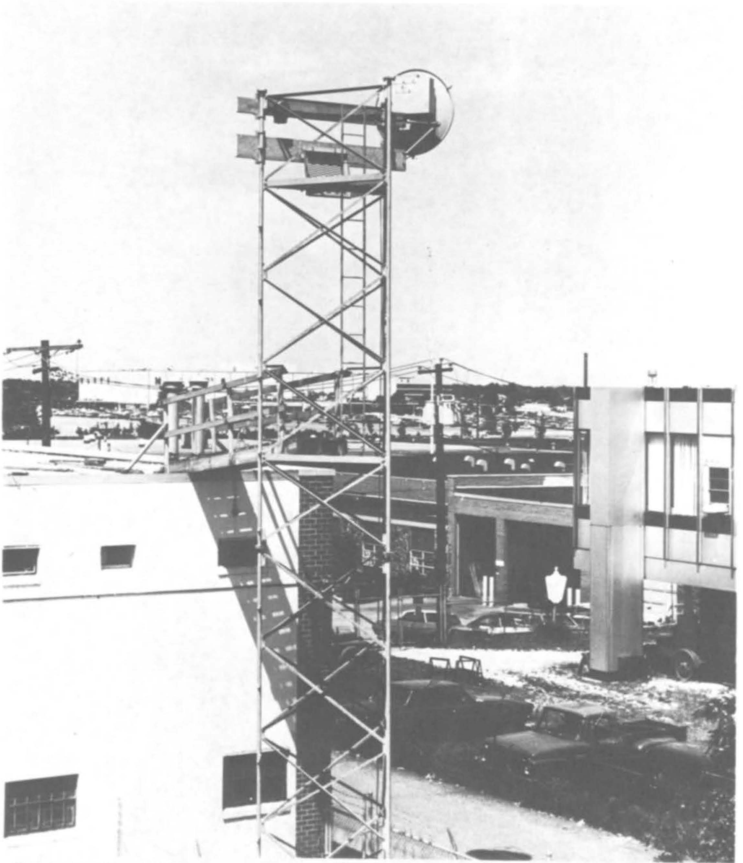
The Laser Link cableless CATV transmitting-receiving terminal in Garden City, NY incorporates quasi laser link concept of antenna and parabolic reflector equipment at top. Back view shows transmitter housing containing modulation and amplification components.
